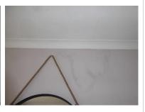
As mentioned above, damp penetration was found causing water staining and damage to the walls/ceilings of the side stacks, where an overhaul to improve water tightness will be required and these stacks, if you do not intend to use them, could be removed in their entirety as they will always be a weak point for damp penetration.
