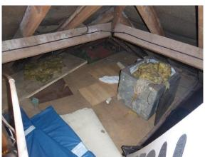
No major defects were noted to the roof structure, but the insulation and ventilation requires improvement.
