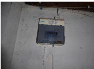
There is a separate consumer unit in the garage, which should comply with regulations, but the lighting was not working and inspection was limited. This should be tested at the same time as the main system.
