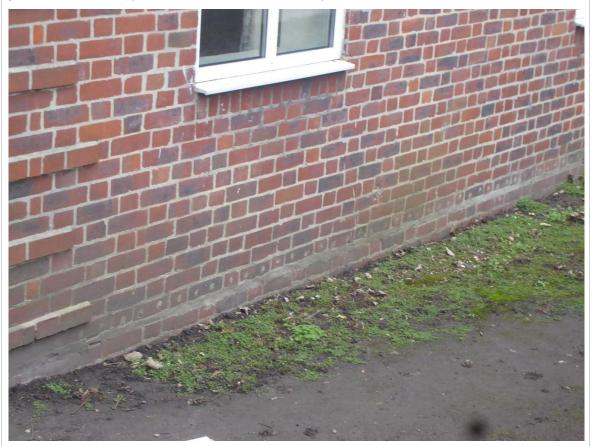
The floors are solid concrete so there is no requirement for underfloor ventilation.
