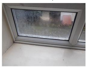
There is black mould growth around the window reveals internally, but these do not show any damp readings and is therefore likely due to poor air management where cosmetic improvements will be required.
